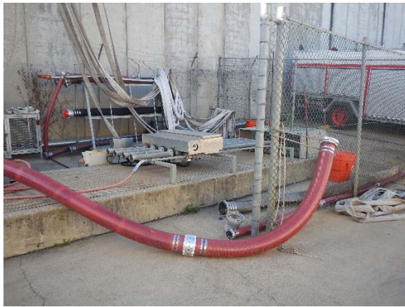
▲ Photograph 1: The pump test area located at the eastern side of the site. AFFF was flushed through the trucks and captured in IBCs. There is a potential for some spills and overflows during this process.
