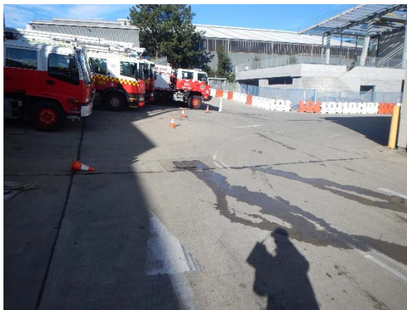
▲ Photograph 3: Facing south in the eastern end of the site. The area was formerly used as fire extinguisher training to the public. The new administration building is being built in the background.
